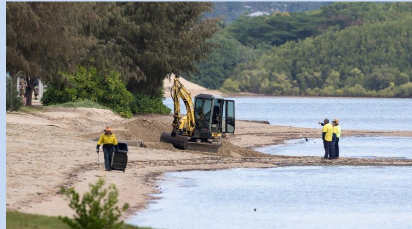
Stormwater sand being spread along Cairns Esplanade – ©Tony Neilson
